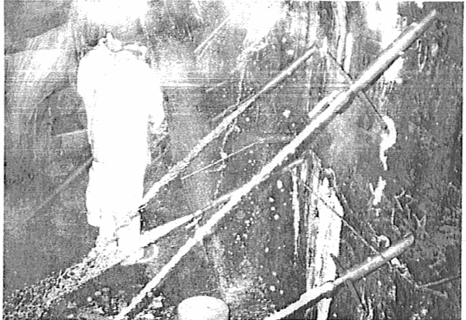
Special packers placed into boreholes intersecting two horizontal lift joints, showing flows prior to resin grouting. The fissures in this section were completely sealed.
